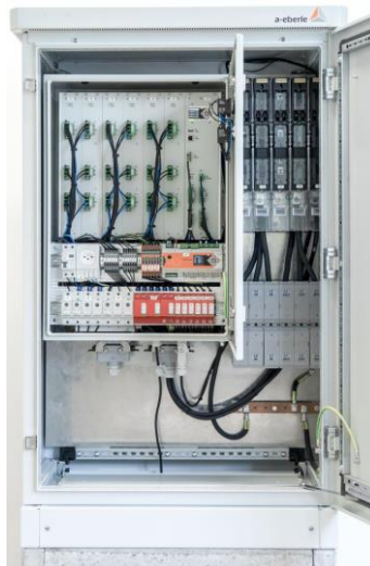
FIGURE 6. Low Voltage Regulator System (LVRSys™) components (70 kVA rating)
